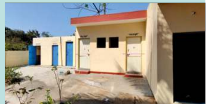
Government School, Byranahalli, Nelamangala Taluk
