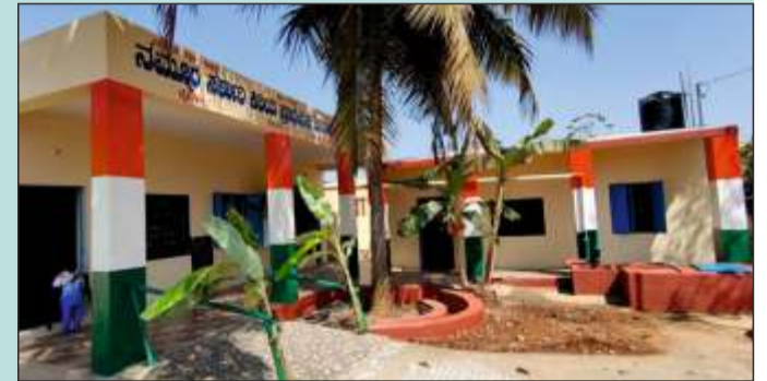
Government School, Byranahalli, Nelamangala Taluk
